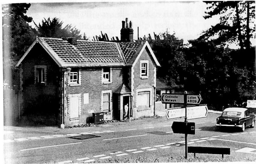
29 The station master's house in dilapidated state at the end of its life, 1966.
