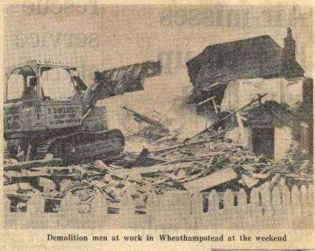
Demolition men at work in Wheatthampstead at the weekend
