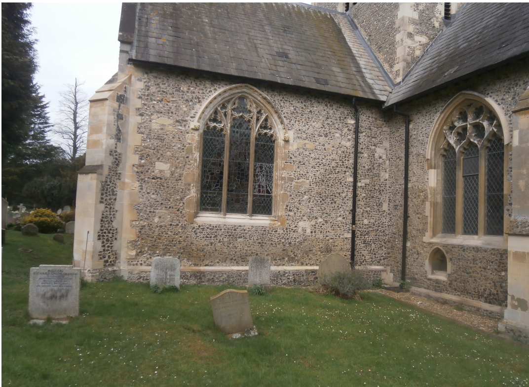
Fig 7. East wall of south transept, showing cut flint and putlog holes with worked stone surrounds
