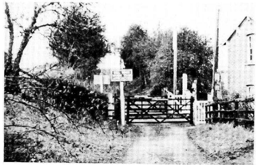
18 The level crossing at the top of Sheepcote Lane. The crossing keeper's cottage to the right.
