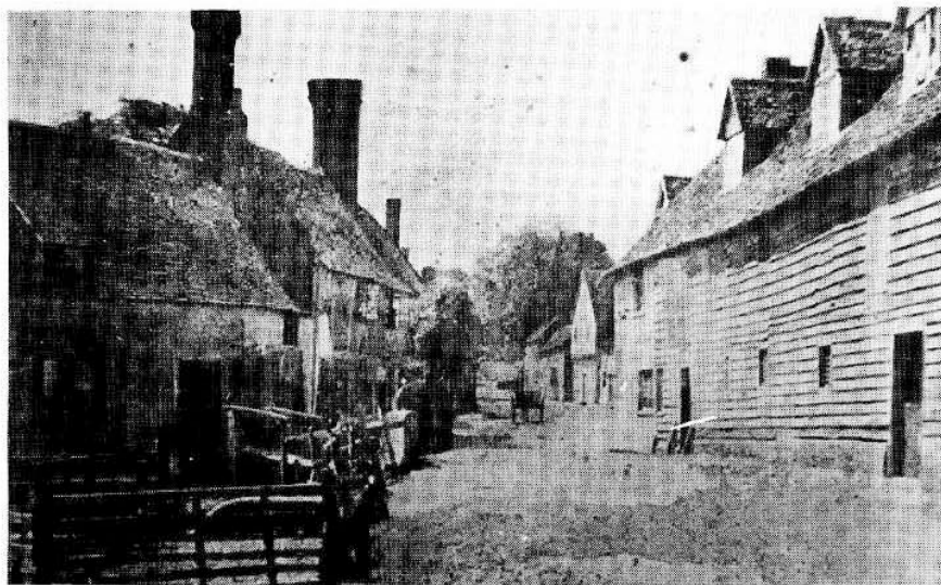
12 An early view of the old boarded mill and The Bull inn, c. 1885, showing the cattle pens.
