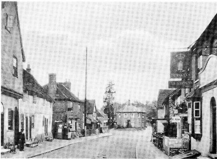
45 The Bell and Crown public house, c. 1920. A good view of the workhouse on the left.
