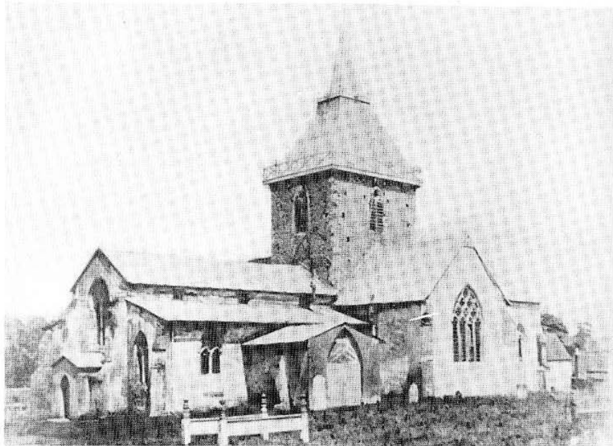
29 A photograph of the exterior of St Helen's church showing the extent of dilapidation before the 1866 restoration.
